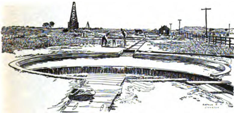
ARTESIAN WELL SYSTEM, RIVERSIDE, CAL. AN AERATOR IN THE FOREGROUND.
